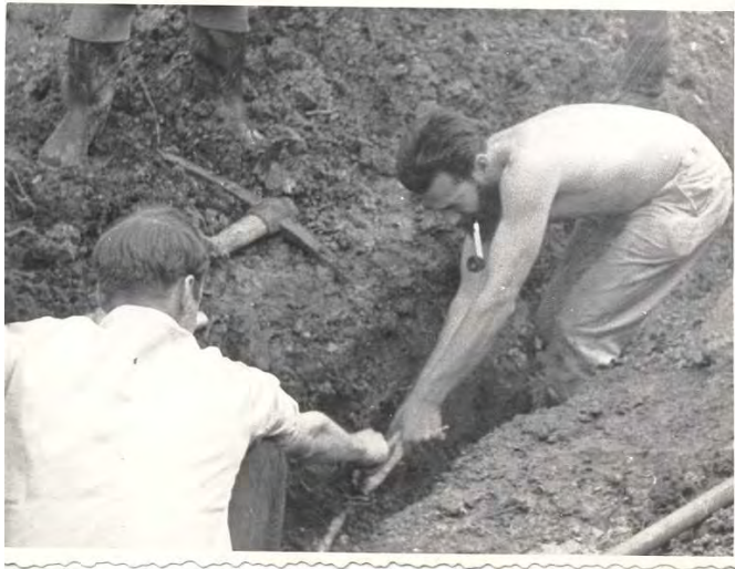
Laying the electric cabling
